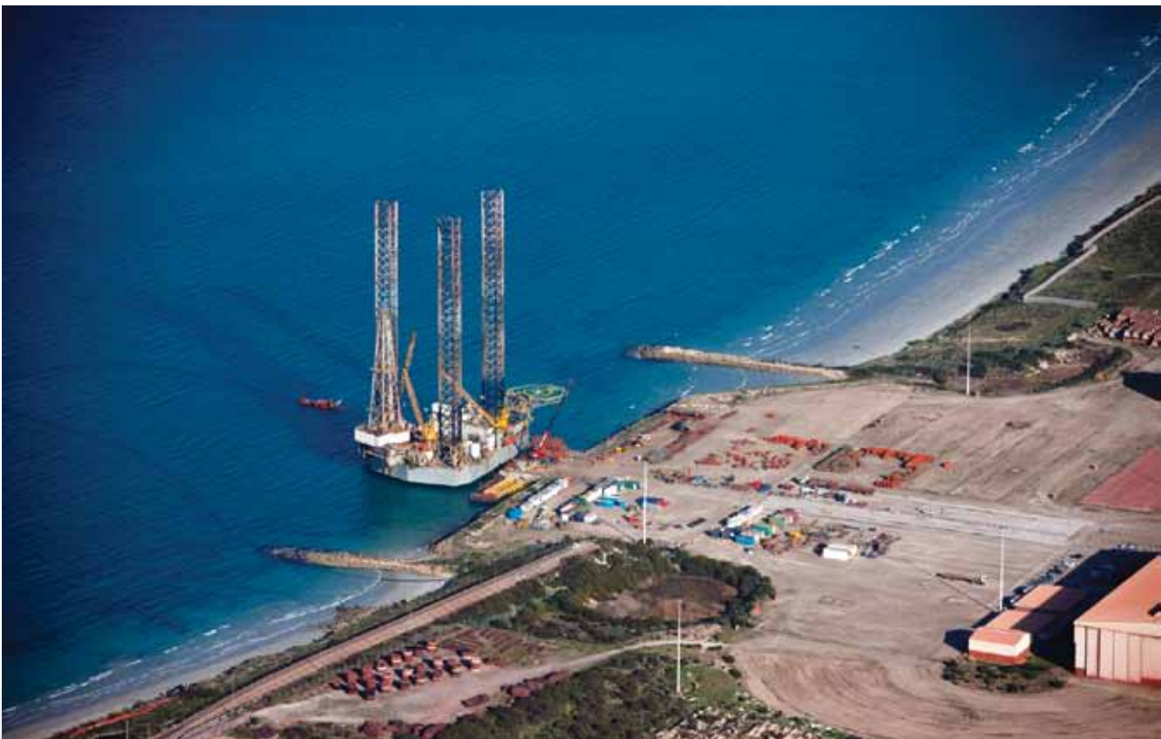
Fig 3.2: (Below) A jack-up rig being serviced off the Moss gas quay from the Offshore Fabrication Yard
